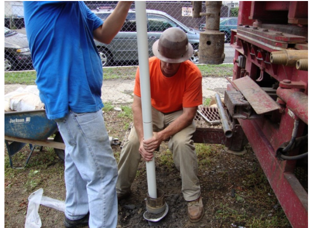
Groundwater Monitoring Well Installation
